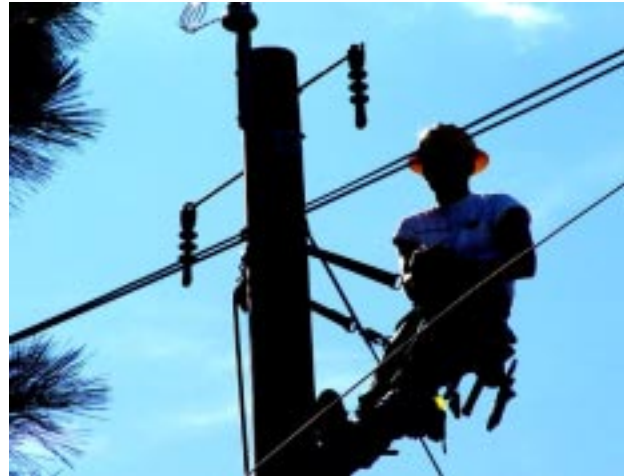
Linemen worked overhead climbing poles on back lot lines
